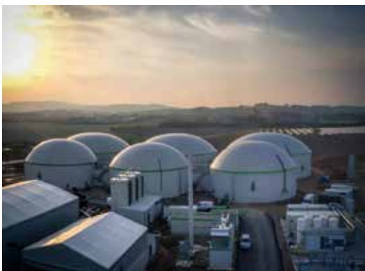
Kanadevia Inova provides integrated on-site waste conversion facilities and emissions reductions.
